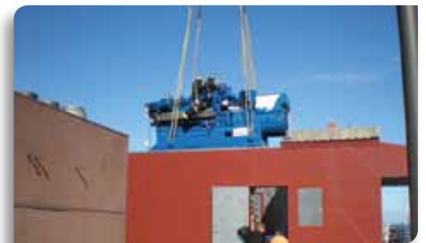
Installing cogeneration into 530 Collins St
