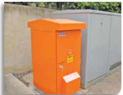
Power Factor Correction Unit
