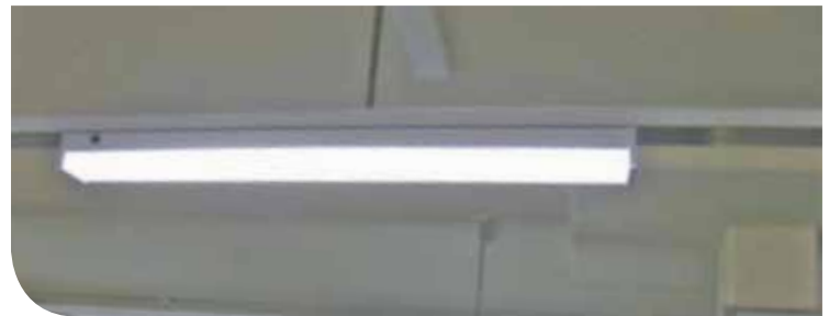
Replaced Light Fitting from 2x36W to 1x37W with reflector and electronic ballast
