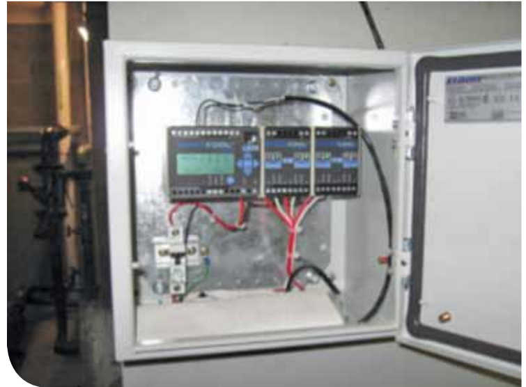
Energy Saving Module on AC Unit
