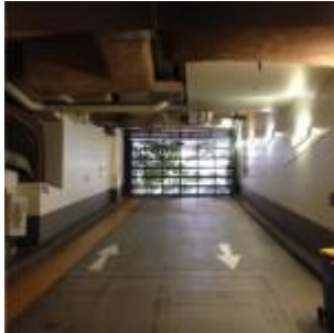
Entry Ramp – Before
